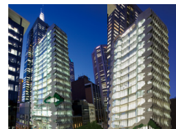
The Office building of the Australian Institute of Architects 41X
